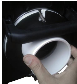
Position Duct Adapter
