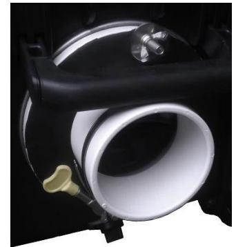
Tighten clamp around duct
